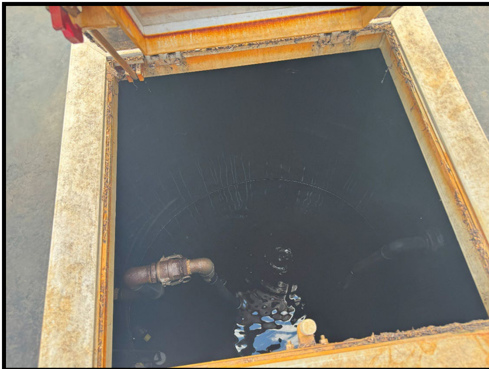
Photograph 4: Leachate at 2/3 full in VLCS-1 sump.
