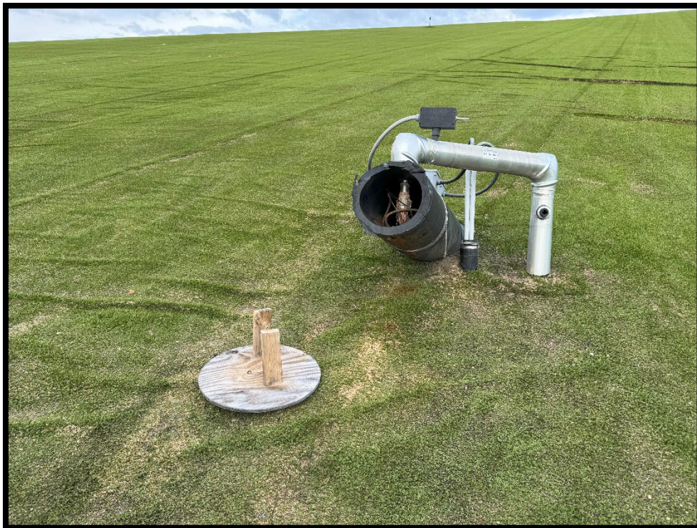
Photograph 8: View of cover removed from LCS-9 sump.
