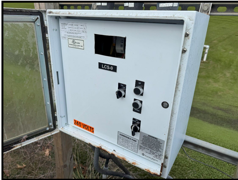
Photograph 7: View of missing display in LCS-9 panel.
