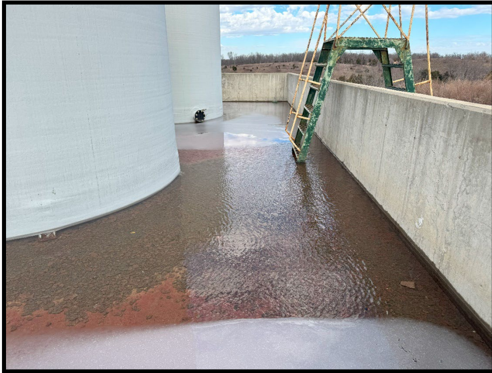
Photograph 5: View of approximately 4-5 inches of stormwater in secondary containment.
