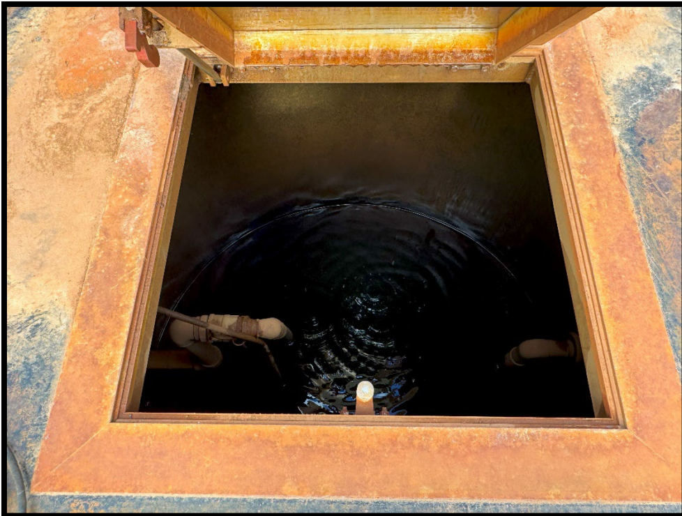
Photograph 2: Leachate at 2/3 full in VLCS-1 sump.
