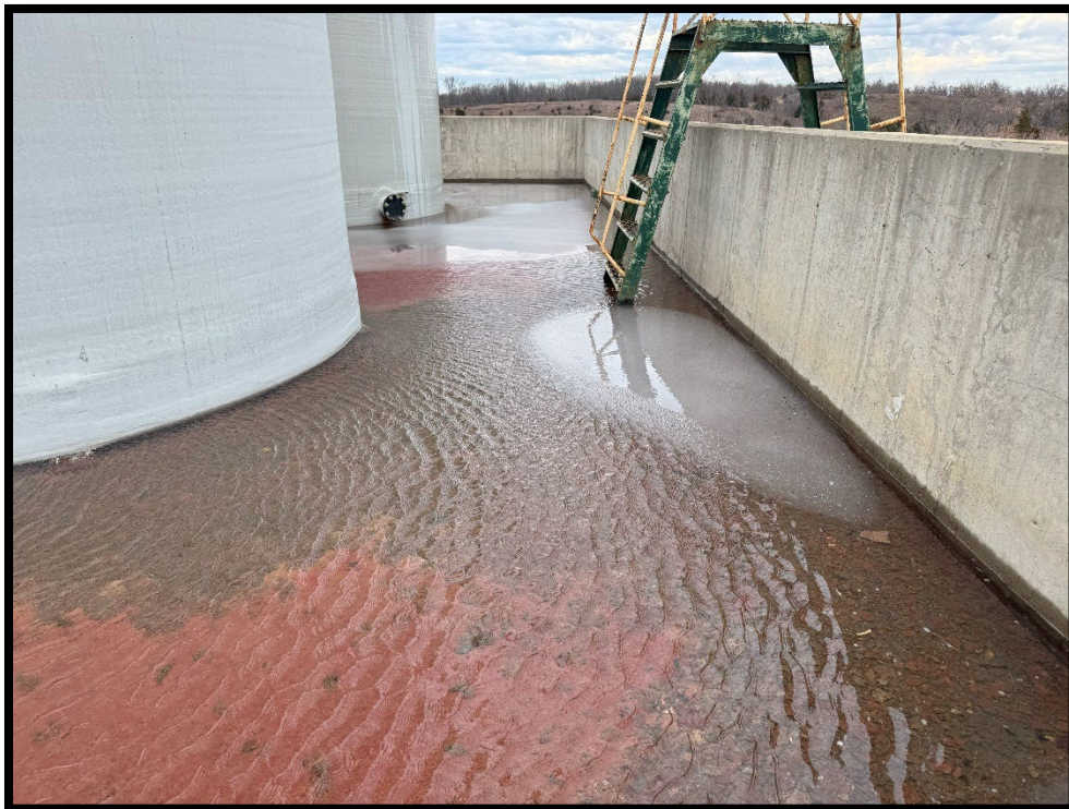
Photograph 6: View of stormwater in secondary containment after release of approximately two inches.
